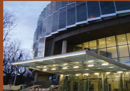
... at The New Criminal Courts, Dublin
