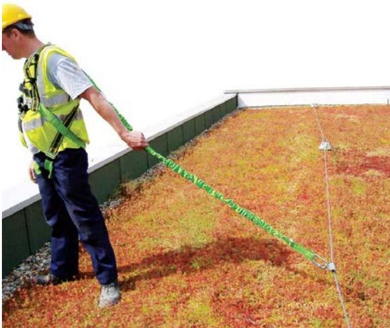
It also important that, where possible, the fall prevention system implemented is a restraint system rather than an arrest system. A restraint system will stop users from falling over a roof edge. An arrest system will allow a user to fall over the edge and will then stop their fall.
